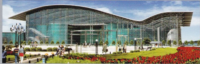
New Ferry Terminal – facilitates comfortable and efficient travel between Hong Kong and Nansha. Frequent 75-minute shuttles connect the two cities.
